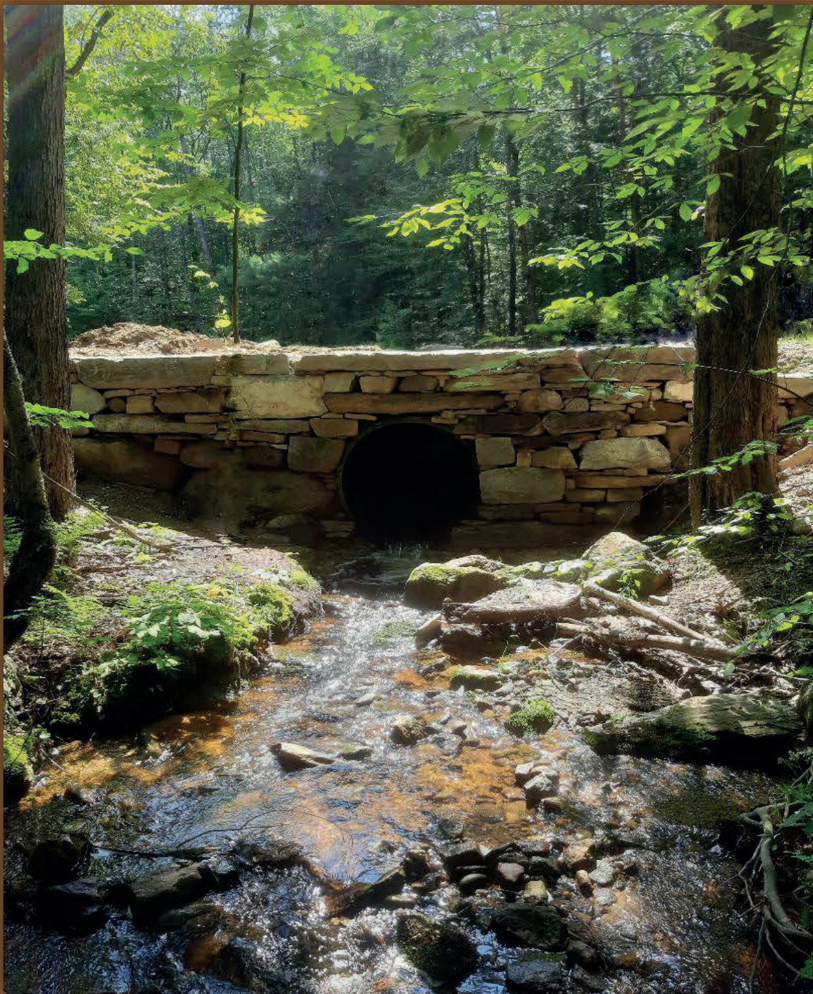
Clough Road culvert stonework project by Dan Schroth & Public Works
